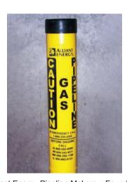
Alliant Energy Pipeline Makers - Found at road crossings, fence lines and street intersections. Markers do not indicate center of pipeline.
